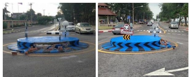
Figure 9 The central island after being smashed by right turning semi-trailer
