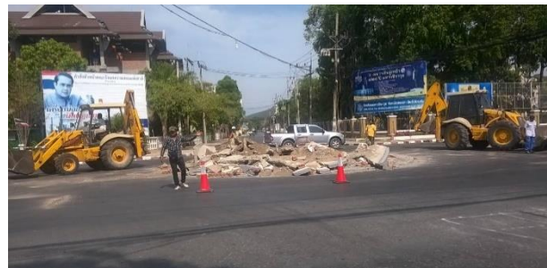
Figure 7 Removal of one of the roundabouts (at location 3) after complaints from residents.
