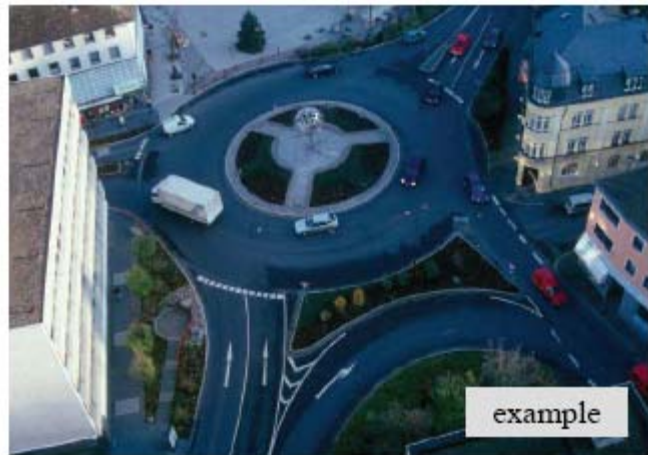
Figure 11. Compact two-lane roundabout inside built-up area, mirrored figures (FGSV, 2006, Brilon, 2005)
